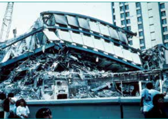
Fig. 8 - Apartment complex collapsed after the 1985 Mexico City earthquake.
